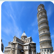
Leaning Tower of Pisa
